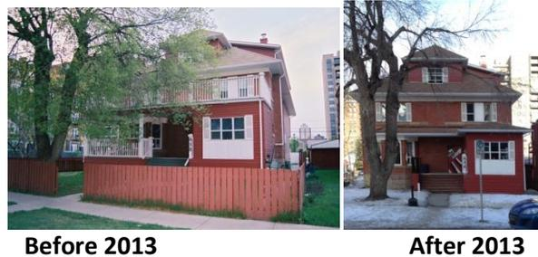
The scope of the work included removal of the fencing, the front and upper story decks and reducing the width of the front steps. Due to the age of the building, brickwork, insulation and roofing were also required.
