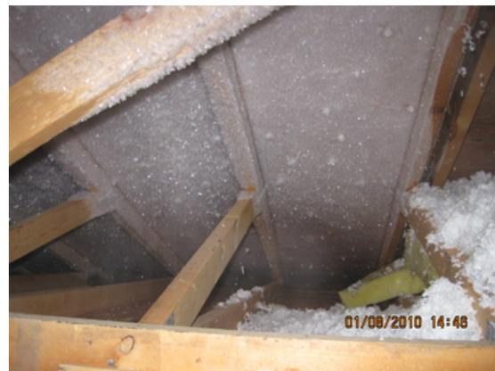
The two main factors in causing attic rain are **Holes & Pressures**. Newer homes have higher insulation levels limiting heat loss while older homes can experience attic rain after adding insulation or a new furnace. Adding ventilation **does not** prevent attic rain.
