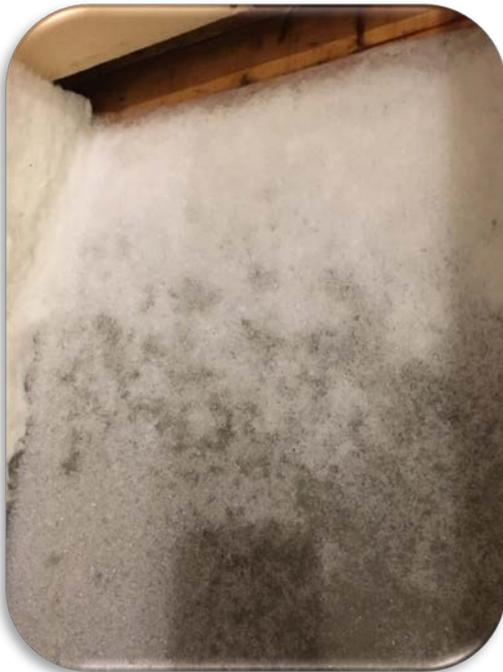
Frost build up (left) can occur across your home, especially in basements. Contrary to popular belief, concrete is not an impermeable barrier and water is capable of passing through. When warm air comes into contact with a cold surface, like a basement floor, condensation occurs.
